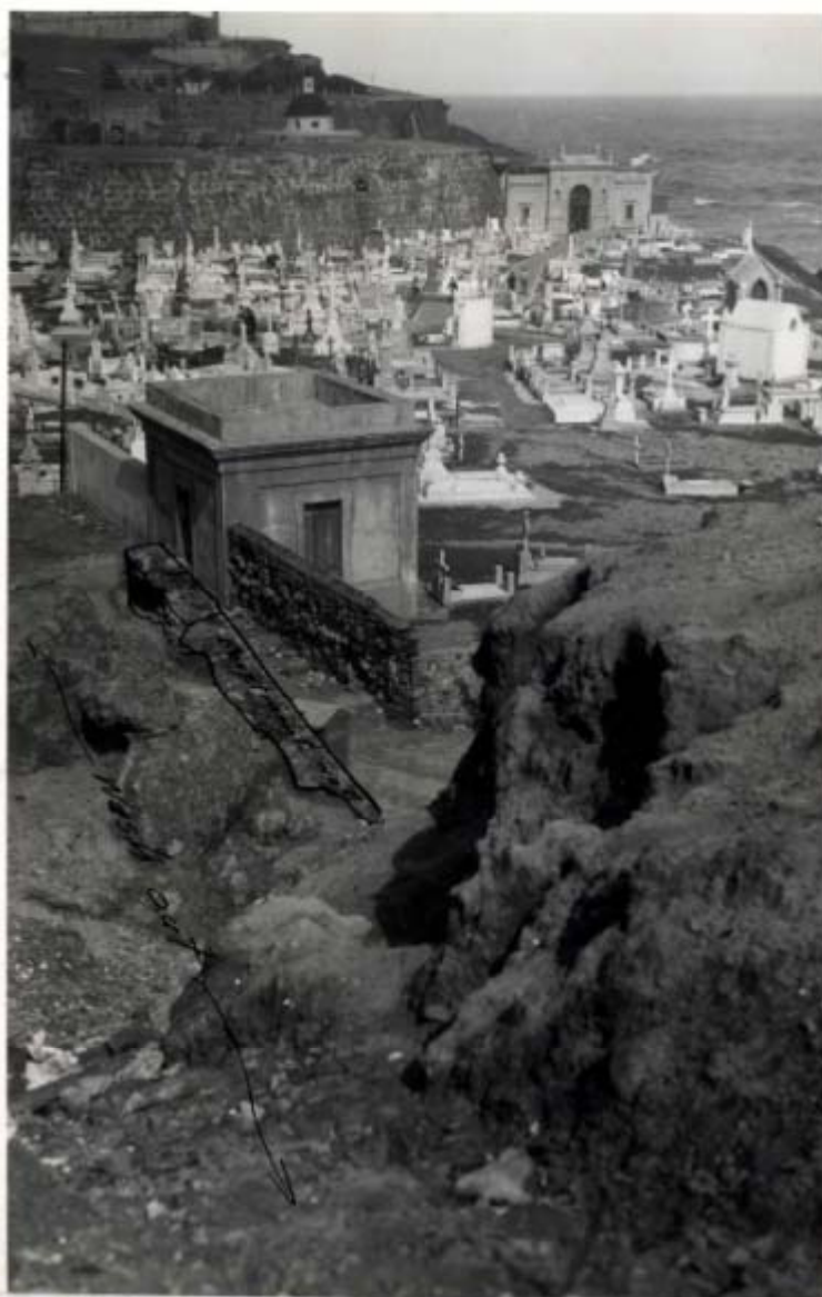
Historical Fortification Walls. San Juan, P.R., Oct.- 1937. (To accompany report from San Juan Office, Mar. 31-1938. Repairs with W.P.A. allotment. F.Y.1938) Item VIII (b) - San Domingo Bastion, North face - looking west, parallel with wall. Shows erosion of back-fill between scarp revetment and bastion wall.
